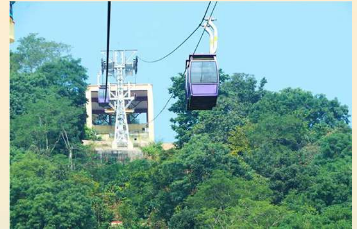
ROPE-WAY AT GANDHI MINAR, HIRAKUD DAM
