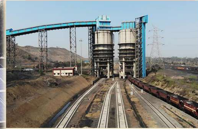
Lingaraj SILO (20 MTPA- Peak Capacity)
