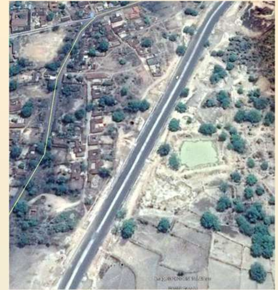
DIVERSION ROAD OF KULDA OCP
