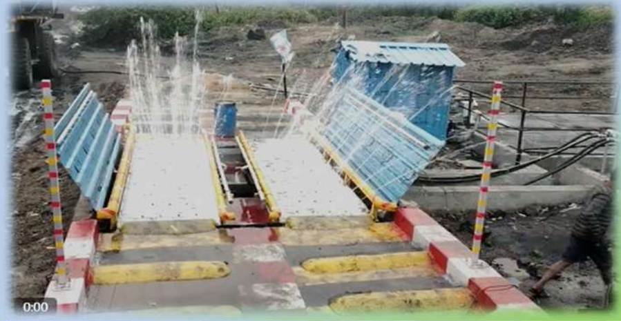
NEW WHEEL WASHING SYSTEM AT JAGANNATH OCP
