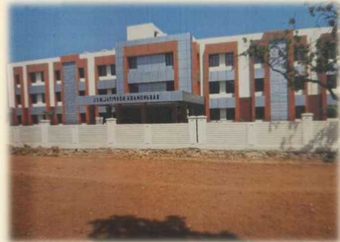
50 BEDDED HOSPITAL AT BASUNDHARA AREA
