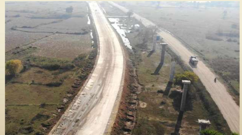
NEW COAL CORRIDOR ROAD AT HINGULA AREA
